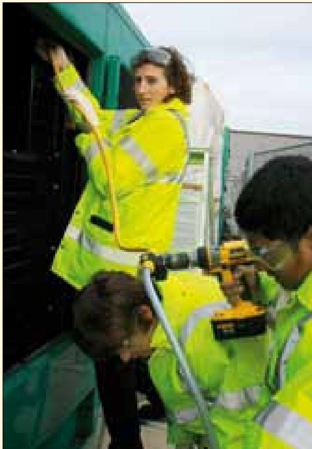
Piers, Chris and Bassam fill the generator
